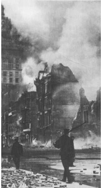
Figure 15 San Francisco Earthquake The fires that caused much of the damage from the 1906 earthquake could not be put out because of ruptured water lines.
