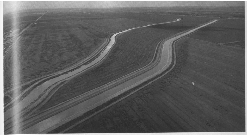
Figure 13 Distributing Water California's State Water Project moves water from the northern part of the state to the south. These aqueducts are near Bakersfield. Inferring What is one disadvantage of moving water through an open aqueduct rather than a pipeline?
