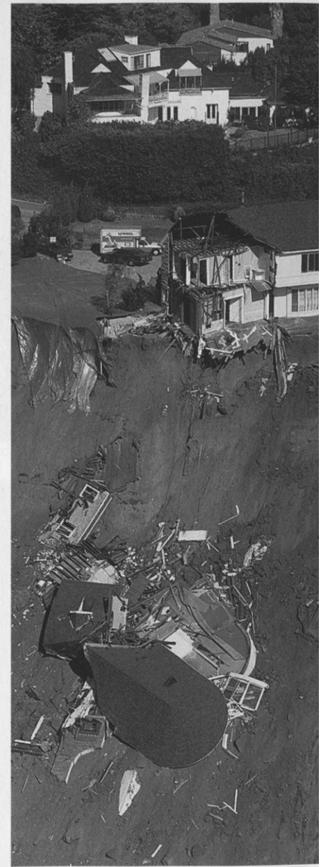
Figure 18 Landslide An earthquake in 1994 triggered this landslide in Pacific Palisades, California. The bluffs had eroded dangerously close to some buildings, making it more likely that an earthquake would cause the collapse shown here.
